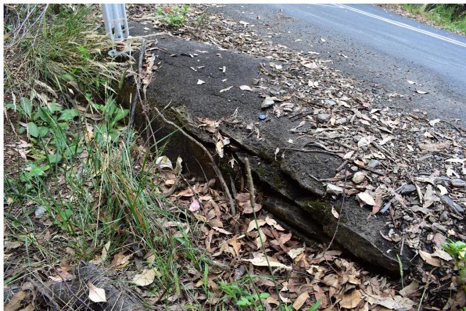
Figure 2 – Example of obscured stonework of culvert inlet along the upward slope.
