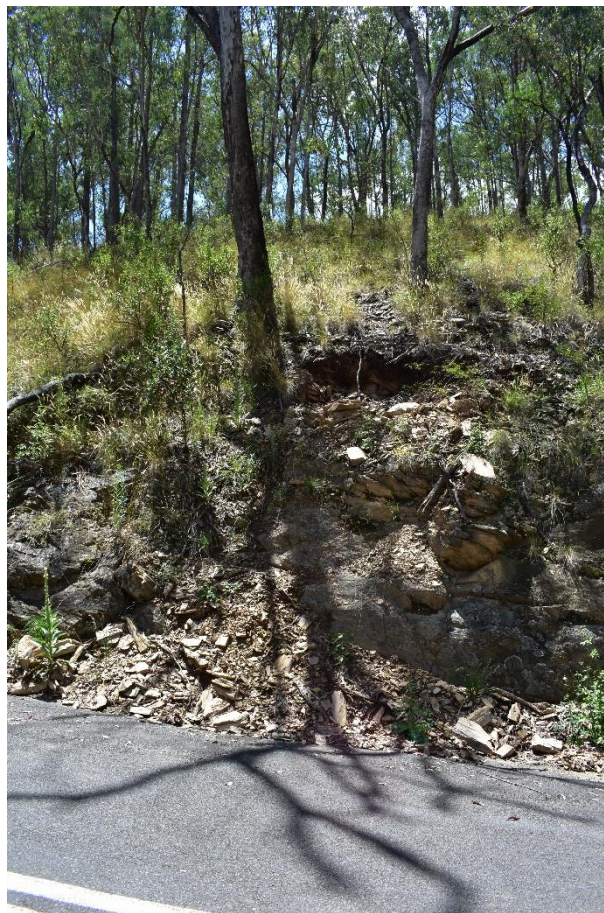
Figure 3 – Evidence of bank collapse/slump on the upward slope in the vicinity of the location of Test Pit 1.
