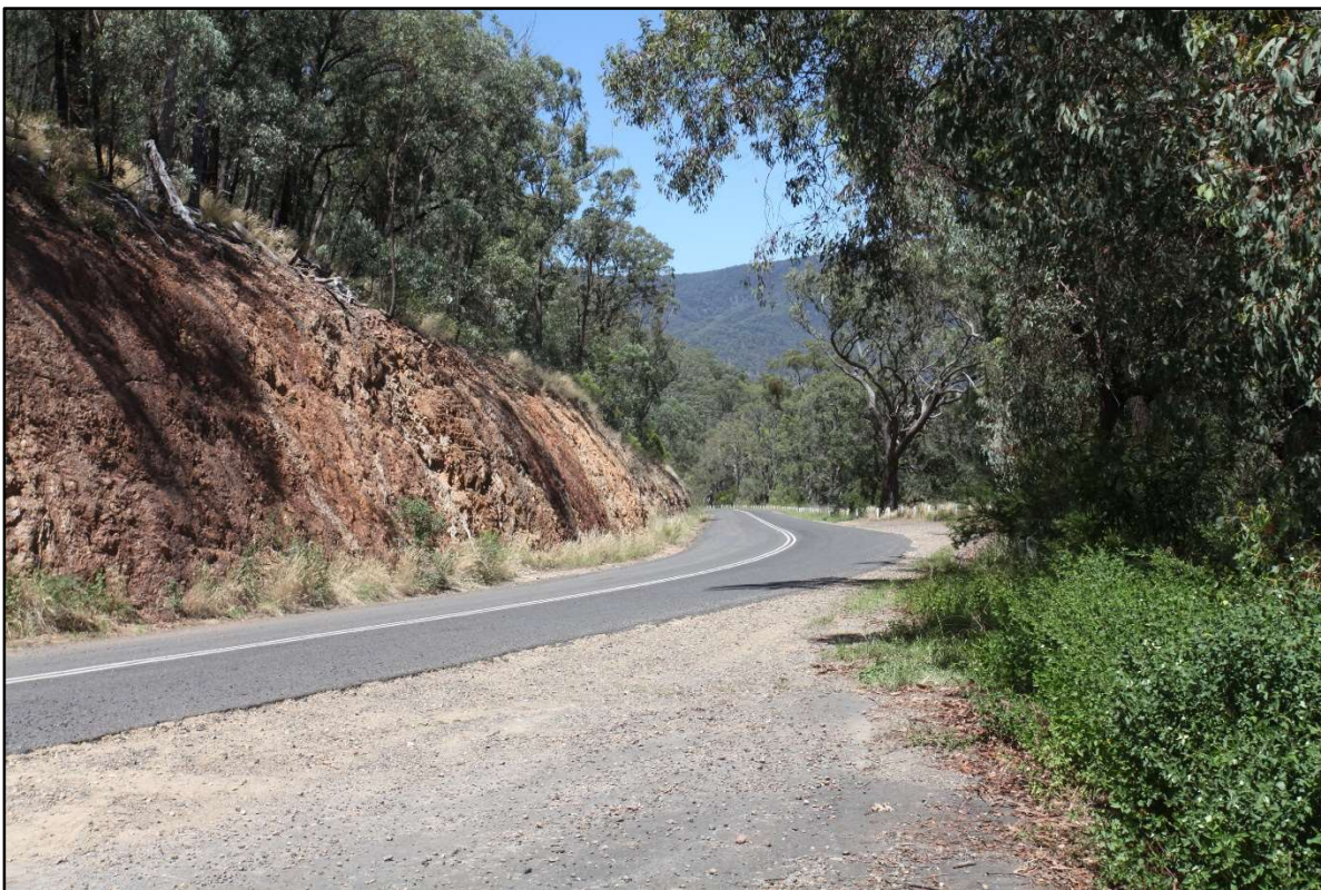
Figure 13: Port Stephens Cutting showing significant cut and fill type construction that would have removed most topsoils
