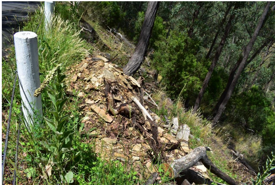
Figure 4 – Evidence of collapse material pushed over upper courses of stone wall at the same location as that shown in Figure 3.
