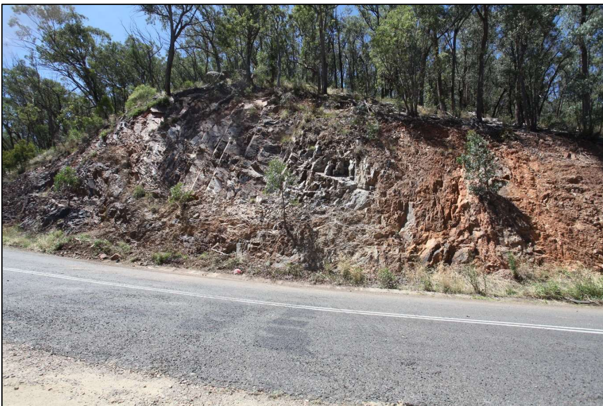
Figure 14: Typical cutting across a small spur/ crest showing low quality 'traprock' type shales
